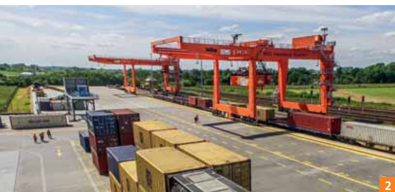
2 PCC Intermodal S.A. is able to transfer containers between road and rail at five wholly owned terminals (in the photo: our Kutno site).
