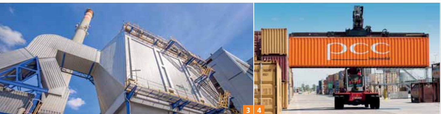
3 The power plant of PCC Rokita SA, a modern CHP cogeneration facility, was further upgraded in 2015 and 2016 with the installation of electrostatic precipitators. 4 The vehicle fleets at the container terminals of PCC Intermodal S.A. were further extended in 2016 through the purchase of a number of new reach-stackers.
