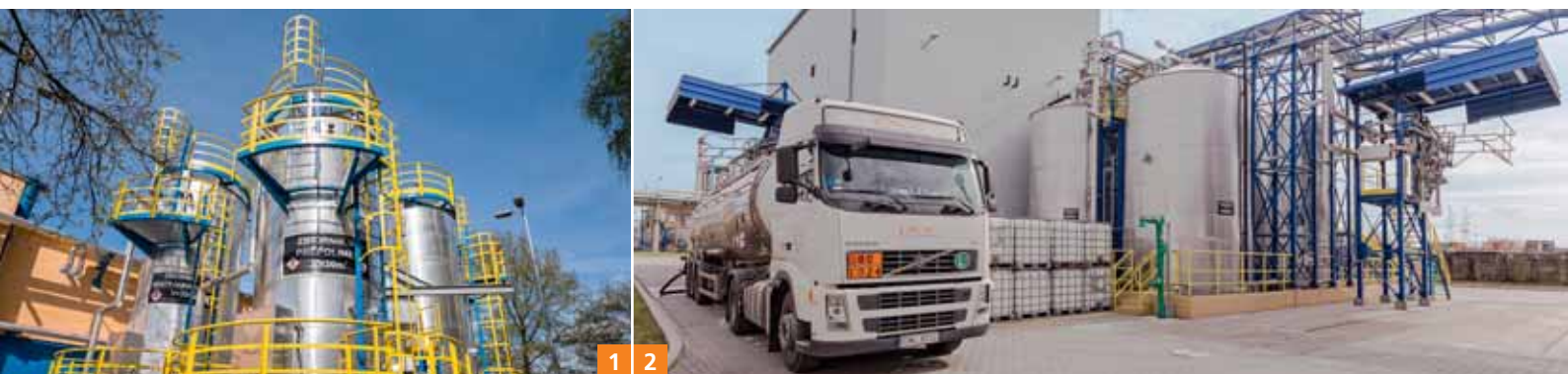
1 Tank farm of the new prepolymer plant of PCC Prodex Sp. z o.o. With an annual capacity of 7,500 metric tons, this counts among the three largest of its kind in Poland. 2 In 2016, PCC Exol SA commissioned a betaine production plant with an annual capacity of 10,000 metric tons.
