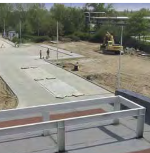
MAY 2010 Construction of the access road with truck weighbridge
