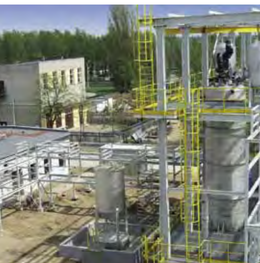
APRIL 2010 Installation of the reactor equipment
