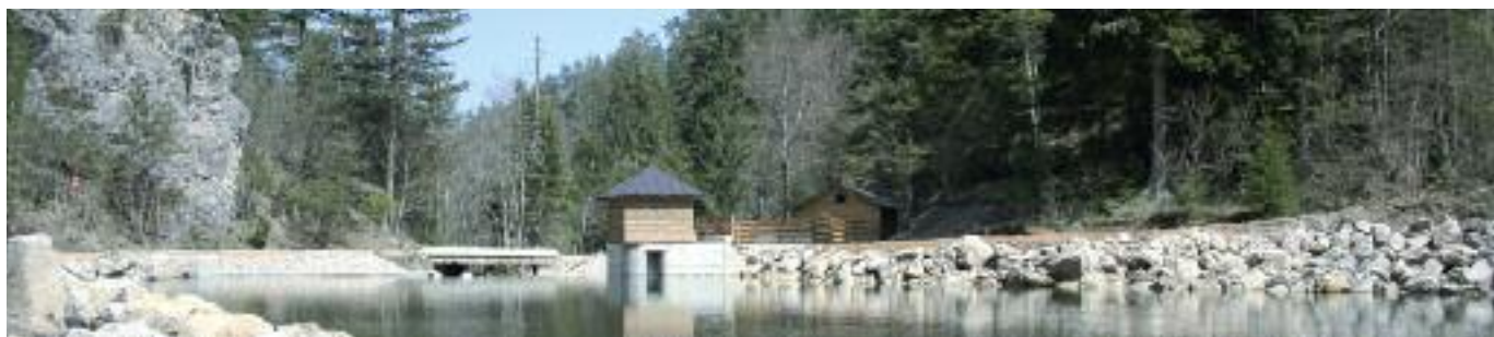
The Mujada small hydropower plant is the first to be completed of a current 18 such climate protection projects in South-East Europe
