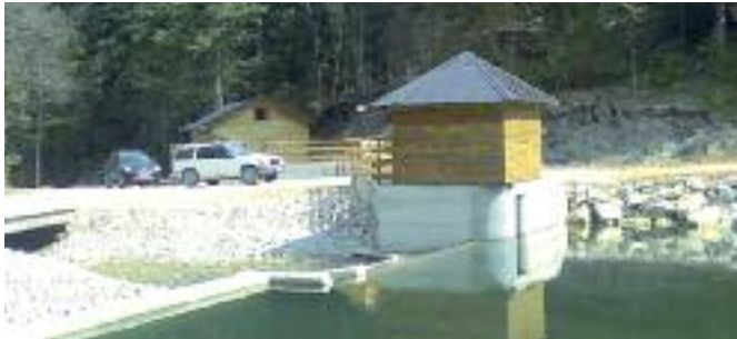
The so-called Tyrolean weir bottom intake system serving the Mujada small hydropower plant
