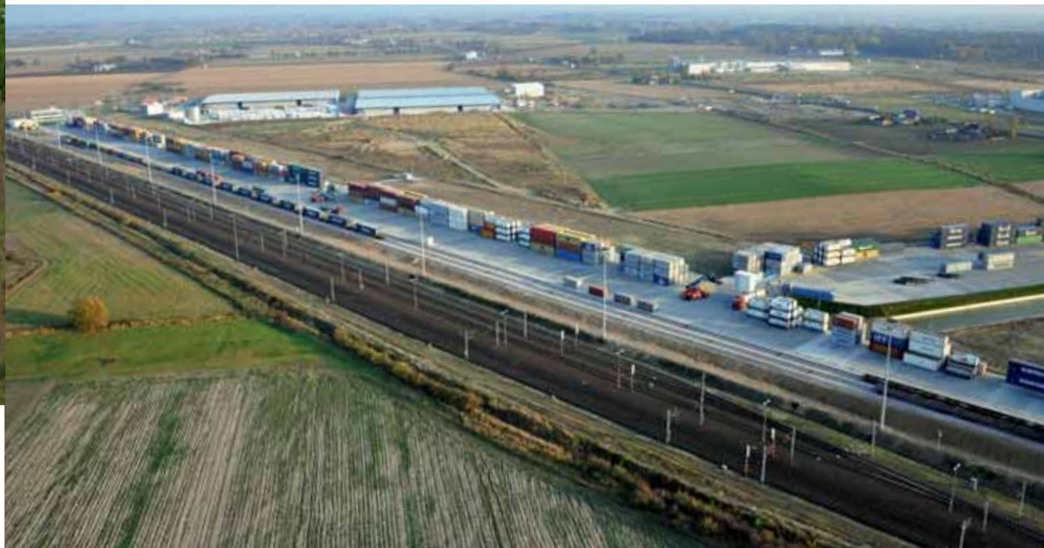
Combined transport terminals of PCC Intermodal S.A. in Frankfurt (Oder) – left – and Kutno – below – which serve in the transfer of containers from road to rail and vice versa.
