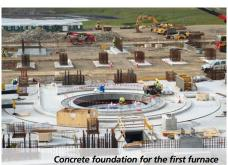
also now almost been completed. Currently, the cladding panels for the side and end walls of the building are being installed. At the same time, work has begun on erection of the first of the two electric arc furnaces. Following the concrete work on the foundations, the rotary gear rim has also now been installed.
