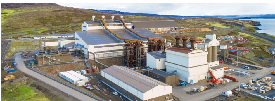
The silicon metal plant of PCC BakkiSilicon hf. in Húsavík (Iceland) resumed production in April with the start-up of the first furnace; the second furnace was subsequently re-ignited in July. Both furnaces are now producing at near-full capacity.
